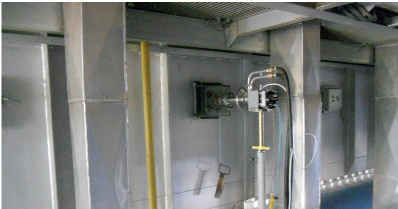
NIR-B 3XR inserted through the steam methane reformer wall.
