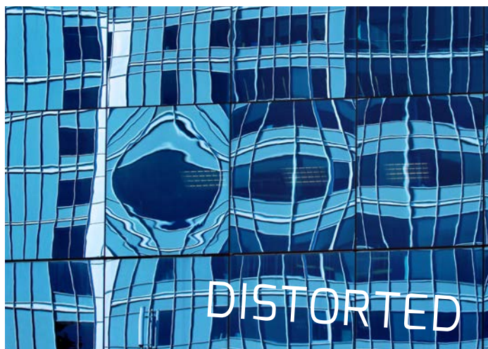
DISTORTION-FREE TEMPERED GLASS – UNIFORM GLASS TEMPERATURE VERSUS DISTORTED GLASS – NON-UNIFORM GLASS TEMPERATURE
